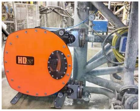
Peristaltic (hose) pumps are able to operate safely, efficiently and reliably in many of the harsh liquidtransfer applications that are prevalent in oil-and-gas production.
