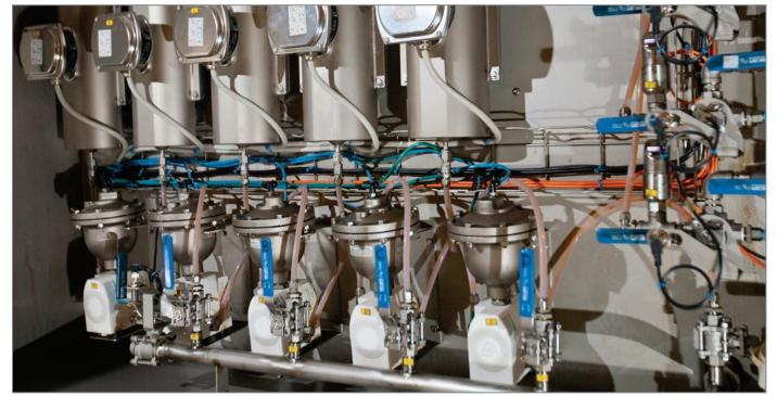
Recently, Technology Unlimited was tasked with fashioning a system for one of Europe's largest animal-feed producers that would inject an enzyme consisting mainly of palm oil onto the exterior of goat feed. The system requirements demanded a dosing pump that would be able to meet all the various operational parameters for temperature, pressure, speed and flow rate.
