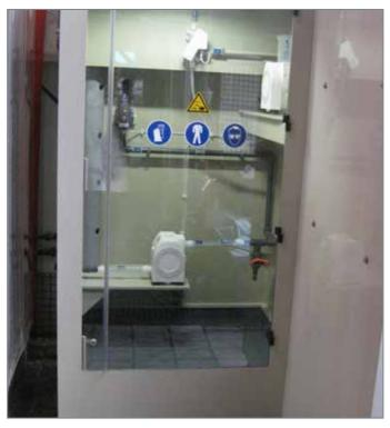
Harsh chemicals can cause compatibility concerns when used with some types of pumps. Almatec® E-Series AODD Pumps can be constructed of plastic materials that are specifically compatible with the chemicals that are being handled, which eliminates corrosion and leak
