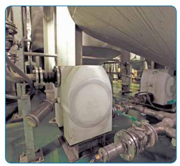
$\label{eq:almatec} \textbf{Almatec}^{\circledast} \, \textbf{E-Series AODD Pumps used for transferring slurry in the solar industry.}$
