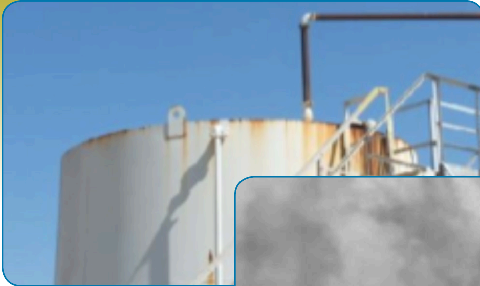
Normal photo of storage tank
