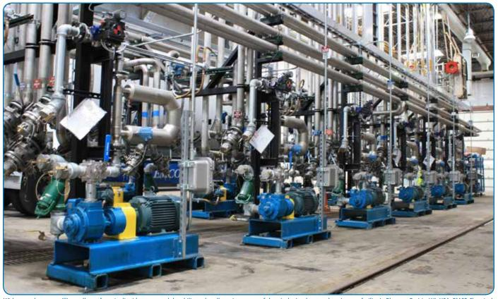
With more than one million gallons of on-site liquid storage and the ability to handle various types of chemicals simultaneously at its new facility in Pleasant Prairie, WI, USA, EMCO Chemical Distributors, Inc., needed to identify and implement pumping technology that could satisfy a wide array of operational parameters. The solution was acquiring 74 GX Series Sliding Vane Pumps from Blackmer®.
