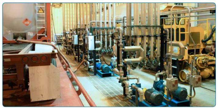
EMCO designed its facility so that tank trucks and railcars could be loaded and unloaded side-by-side. Adding to the efficiency of this design are a series of Blackmer® GX Series Sliding Vane Pumps.
