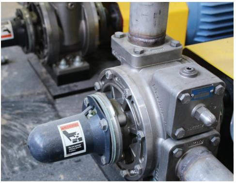
Pumps used during the DEF production and loading/unloading process must be compatible with DEF's unique characteristics. This is why Brenntag North America relies on STX-DEF Series Sliding Vane Pumps from Blackmer<sup>®</sup>.
