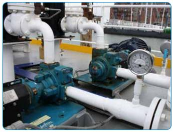
Harbor Fuel 1 is outfitted with Blackmer GX & X Series pumps, a 2-1/2-inch model for highcapacity fuel transfer, and a 2-inch version for operations that require lower flow rates.
