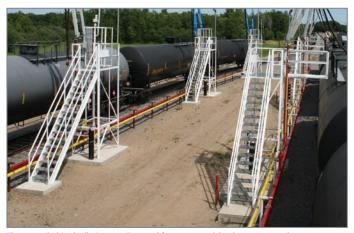
The expanded Rockville Propane Terminal features 10 rail-loading towers and 16 propane-storage tanks with a combined storage capacity of 620,000 gallons. A second loading island was also built, doubling the number of transports that could be loaded in any given day.
