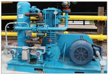
The Blackmer® compressors are ideal for the Alliance terminal's needs because they feature single-stage, oil-free operation and have been designed specifically for propane transfer and vapor recovery.
