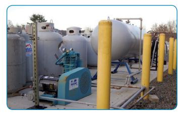
Bluhms installed a designated vapor-recovery pad in 2008 to capture all of the vapors from any tank being serviced. Bluhms estimates that they've recovered 40,000 to 50,000 gallons of gas since installing the system.
