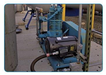
The LB Series Reciprocating Gas Compressor from Blackmer is the focal point of Bluhms Gas Sales' vapor-recovery system.
