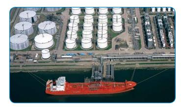
In short, any liquid that can be transported in bulk be it by ocean-going tank ship, barge, railcar, tank truck or pipeline—at some point in its life is stored and transferred at a liquid terminal with the storage tank operating as the interface between the various modes of transportation.
