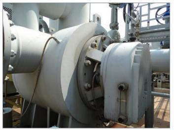
Blackmer S Series Triple Screw Pumps are made to handle clean lubricating fluids without solid content across a wide range of viscosities, temperatures and pressures. This method of operation delivers smooth, constant product flow with low noise and high levels of energy efficiency, which are critical concerns in oil-and-gas fluid-handling applications.
