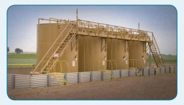
When crude oil is gathered and stored in a tank battery the chance for vapor escaping is very high. Vapor-recovery systems that feature Blackmer Oil-Free Reciprocating Gas Compressors can capture these vapors providing increased safety and additional revenue for the producers.
