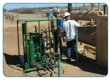
Non-lube reciprocating gas compressors help control condensate that may form inside the compressors. Blackmer compressor designs provide a means to control small amounts of condensate by collecting it in an area of the compressor called the distance-piece compartment.
