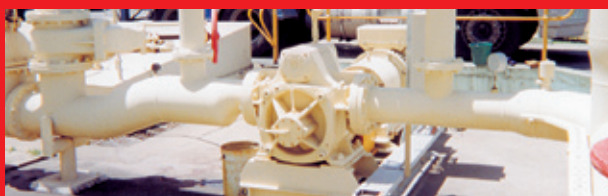
Bunkering / unloading molasses
