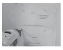
2. Drill holes for the wall anchors with 5/16" drill bit. Install anchors.
