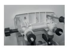
7. If not using wall bracket, fasten unit to wall using the top two mounting holes located on the cabinet back.
