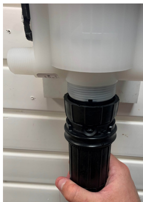
Step 8. Replace lower end assembly.
