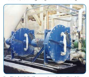
Abaque™ Series Peristaltic (Hose) Pumps possess the operational versatility to reliably handle a wide array of fluids in paint-and-coatings manufacture, from viscous slurries to water-thin liquids.
