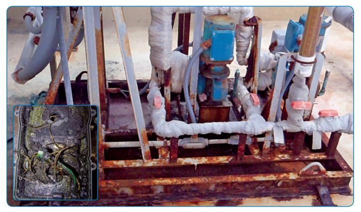
Acids do not discriminate when attacking equipment that has not been properly designed for its handling. As viewed above, for example, a skid treated with inadequate coating or a pump misapplied for acid-feed use (inset) all display the effects of acid corrosion.
