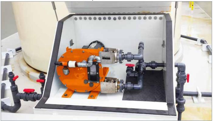
Peristaltic pumps are ideal for various chemical-handling applications in wastewater treatment because their simplistic design and operation allows them to reliably handle both viscous and abrasive chemicals.
