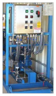
Hydraulically actuated diaphragm metering pumps are a leading technology of choice for wastewater-treatment plants because they can handle the harshest chemicals, can pump against higher pressures, offer highly repeatable dosing accuracy and have been designed for 20 year of service.
