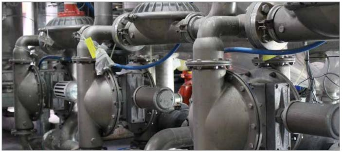
Wilden® Original™ and Advanced™ AODD pumps are the perfect solution for Havo thanks to their ability to handle high-viscosity liquids. Additionally, Wilden pumps feature a redesigned liquid path that reduces internal friction for maximized flow rates and pumping efficiency.
