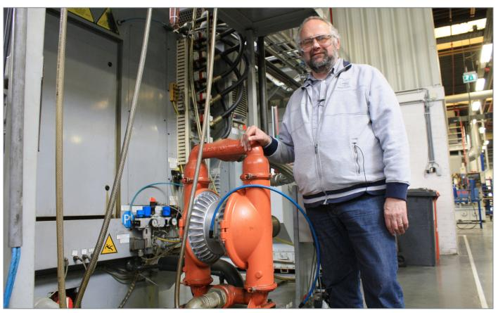
John Bollebakker is the Manager of Maintenance and Facilities at Chromalloy. For more than 15 years, he has trusted Wilden® Original™ Series AODD Pumps to reliably transfer the cooling fluids that are used to keep the repair and refinishing machinery operating safely when servicing the gas-turbine engine components used by commercial airlines and other operators.
