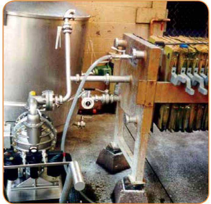
The operational advantages of using AODD pumps in winemaking processes are many, including easy to clean and maintain; gentle handling of delicate fluids; capable of moving large volumes; seal-less design; and portability.
